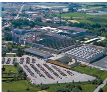
Stiebel Eltron's plant in Holzminden, Germany.
