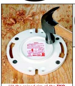
Hit the raised rim of the **TKO** until the knockout cracks loose.
