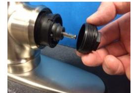
5. Grab the metal stem sticking up and lift the cartridge out of the faucet.
