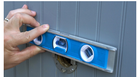
Step 4 cont'd: Ensure mounting bracket is level
