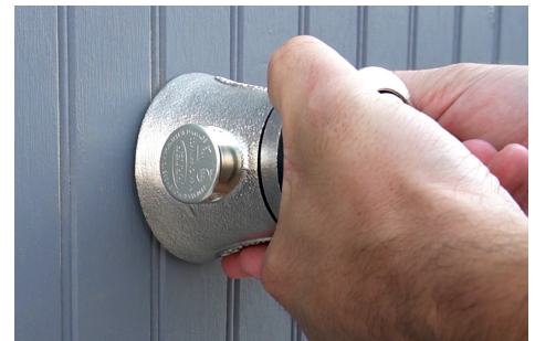
Step 5: Vacuum breaker is at the 9 o'clock position, and the spout is at 3 o'clock
