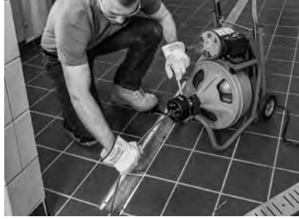
Figure 15 – Operating K-400 with AUTOFEED
