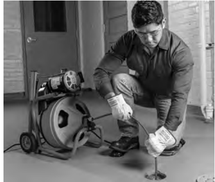
Figure 13 – In Operating Position, Manually Feeding Cable
