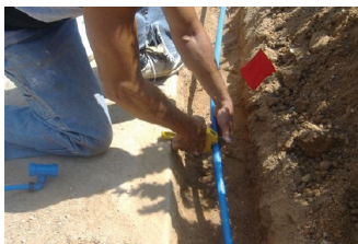
2. Cut-into the lateral line
