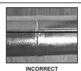
Figure 3.3 - Make sure the seams are not aligned to prevent unintentional disconnection.
