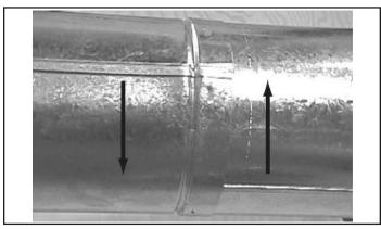
Figure 3.8 - Rotate Seams for Disassembly
